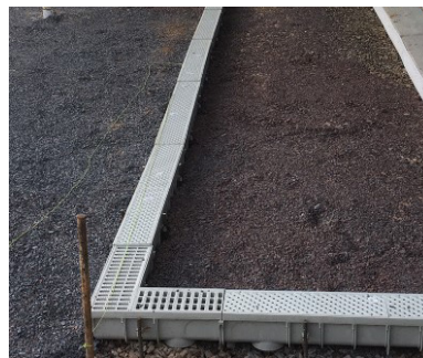
Photos: Nor-Gwyn Pool Commission project to install new deck drainage around the entire perimeter of the main pool along with replacement of the decking and lighting around the main pool.
