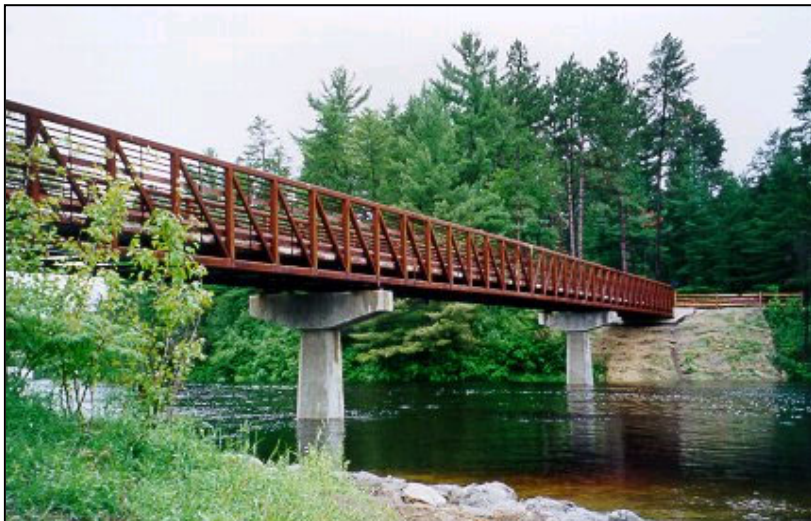
Example of Independent Trail Bridge
