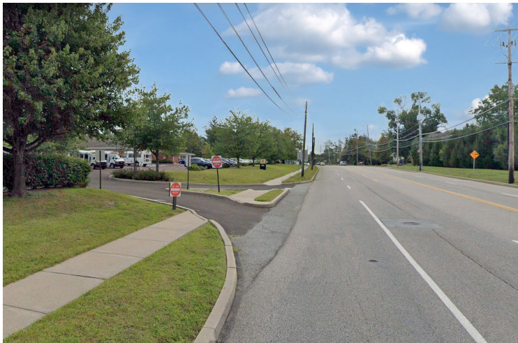
Segment 3 replaces the sidewalk on the north side of Sumneytown Pike with a shared-use side path. Signage and pavement markings will be placed at driveway entrances
