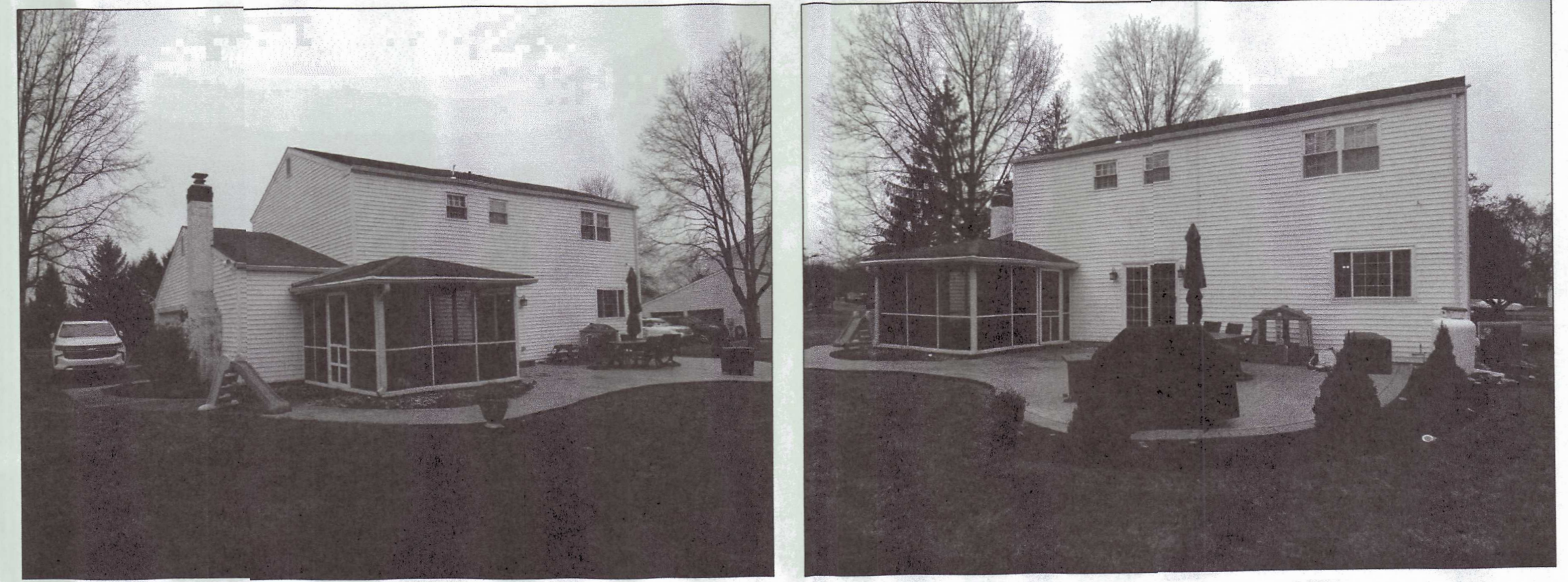
EXISTING CONDITIONS PHOTOGRAPHS NOT TO SCALE
