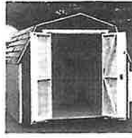
Doors are reinforced with 2" x 4" bracing.
