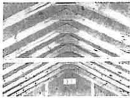
Collar ties are used on all buildings over 18' long.
