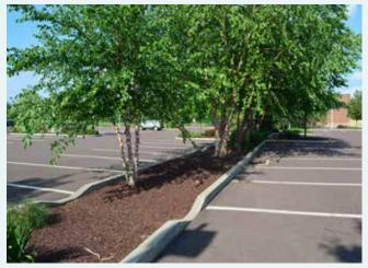
Strategically placed depressions in the curb around parking lot islands can allow runoff to flow into the landscaped area where the stormwater can be infiltrated back into the ground and support the growth of the landscaping.
