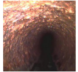
The inside of an iron pipe, that has developed a layer of scale that can snag paper and cause clogs.
